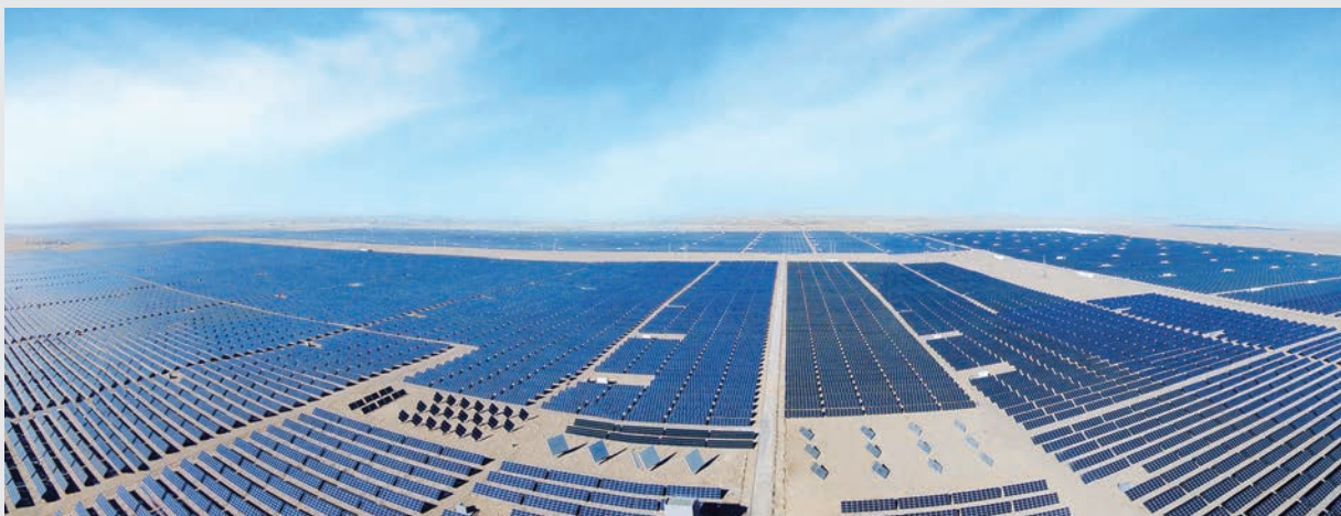
Digital and smart PV power station
