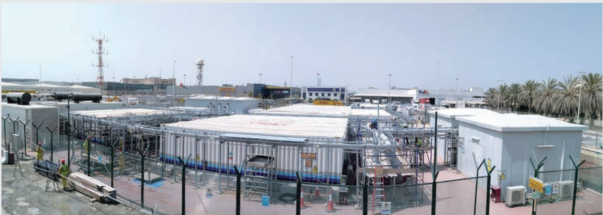
The data center at Dubai Airports
